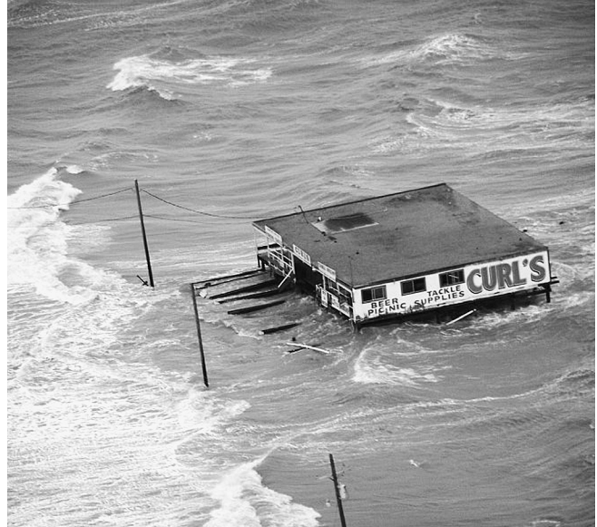
Sea surge from Hurricane Ike overtakes the Bolivar Peninsula bridge near Galveston, Texas, September 12, 2008.
